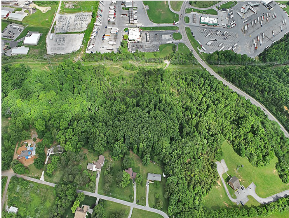
Rooftops (in Farragut) Just South of Parcel
