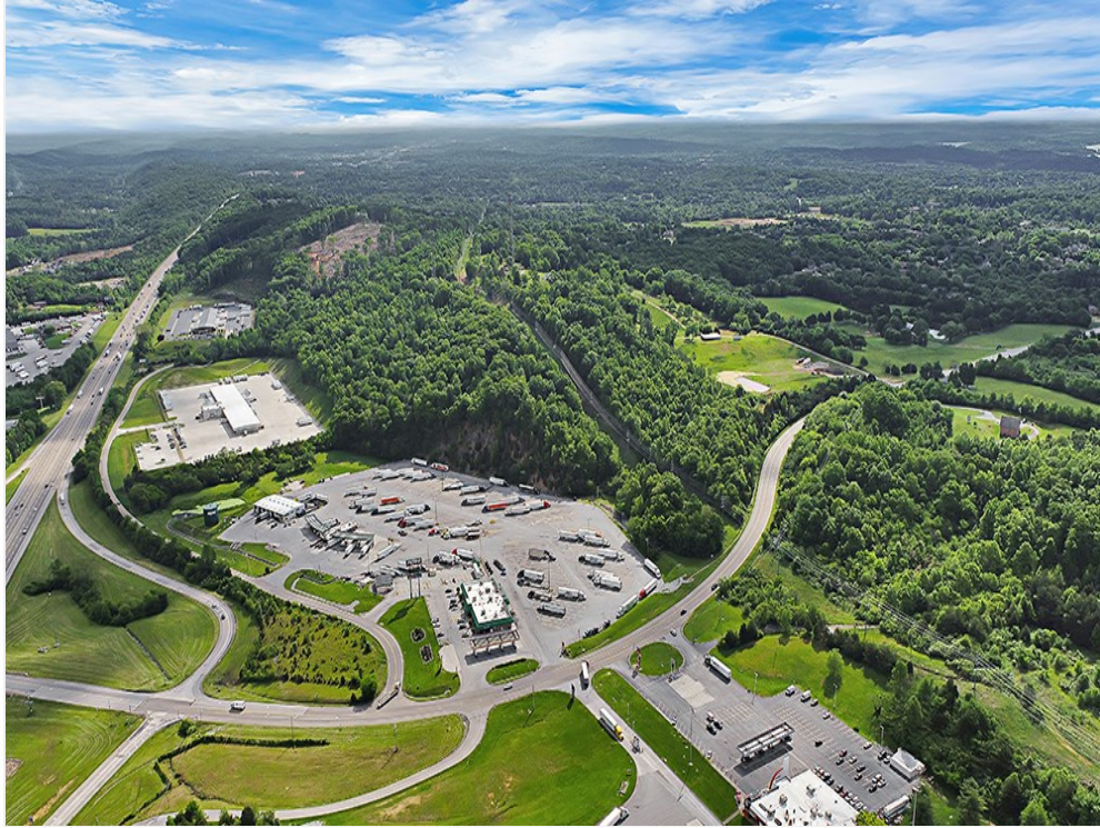
I-40/I-75 Exit (south side ramp)
