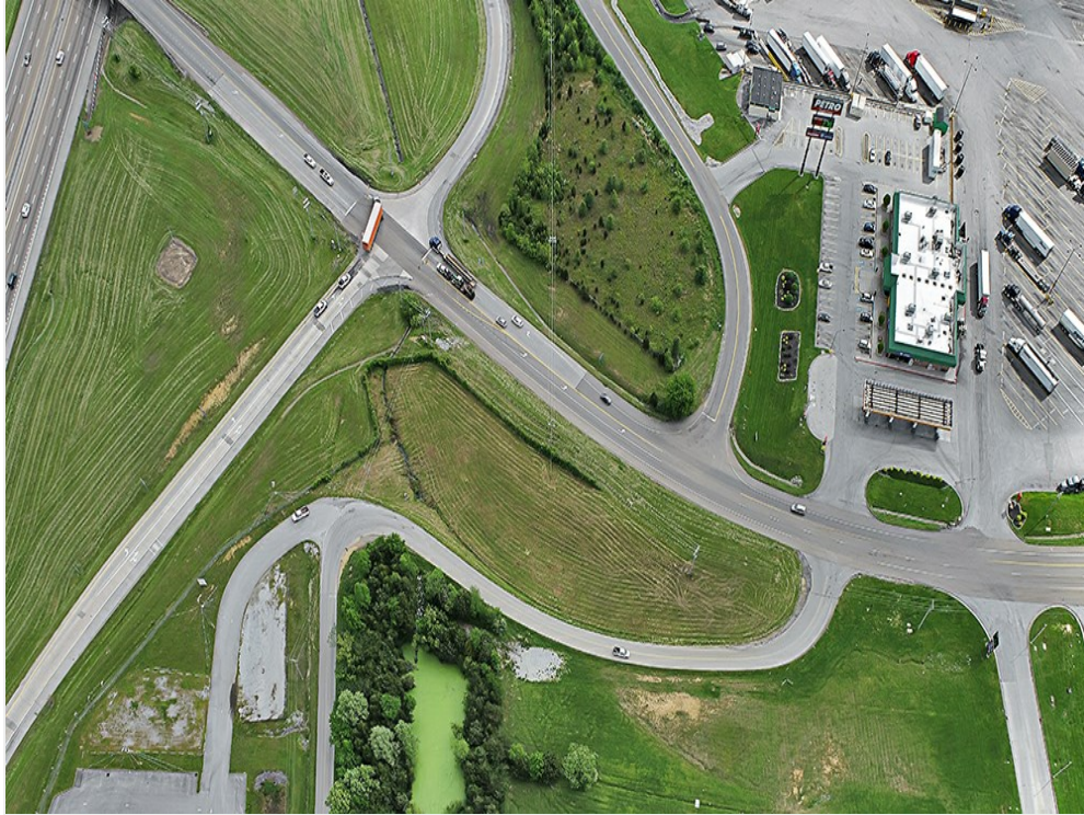
Busiest Truckstop Exit in USA -Cleared Level Ready
